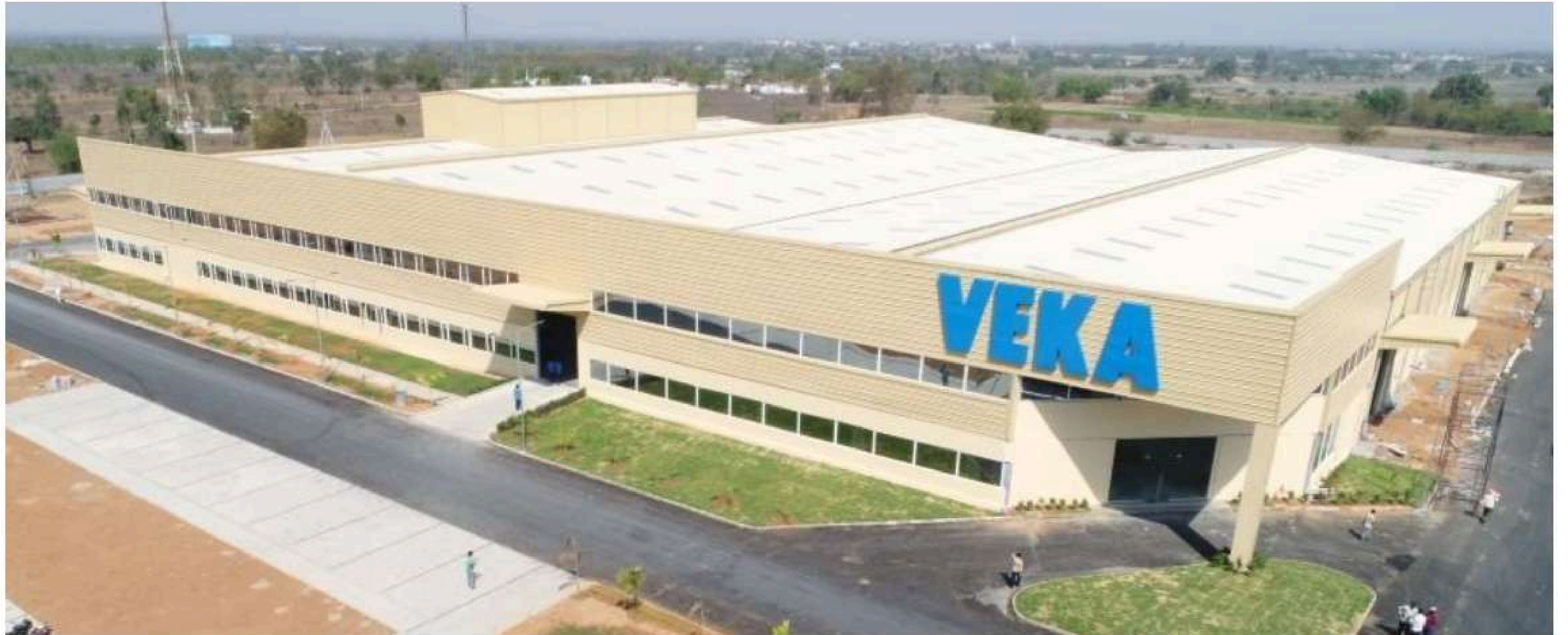
PRODUCTION FACILITY NCL VEKA, HYDERABAD
